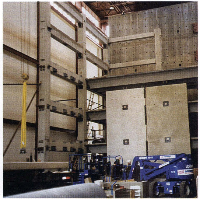
Fig. 4. TCY frame and wall panels under construction.
